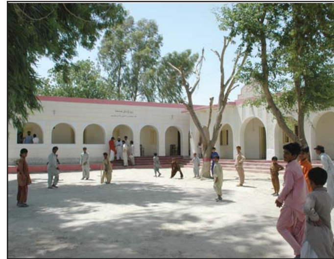
Partially Damaged Renovated School
